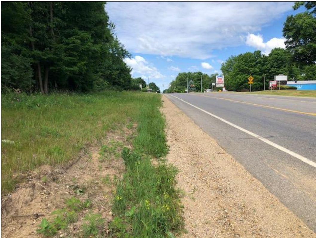
Figure 9. Road right-of-way on the south side of Red Arrow Highway; note graveling and grading.
