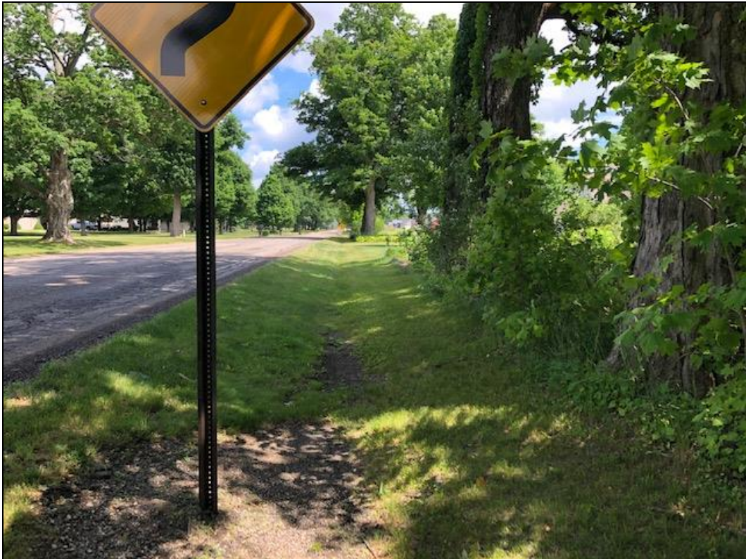
Figure 11. Road right-of-way on the east side of Co Rd 652 St; note ditching.
