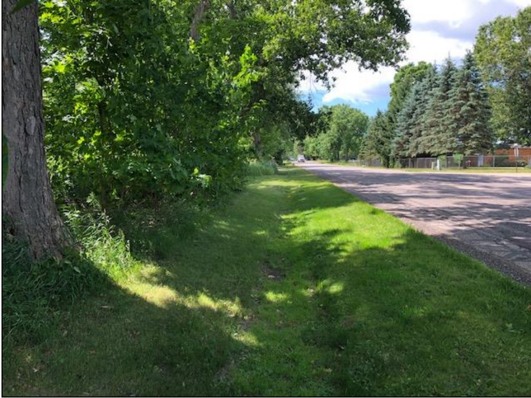
Figure 10. Road right-of-way on the west side of Co Rd 652 St; note ditching.
